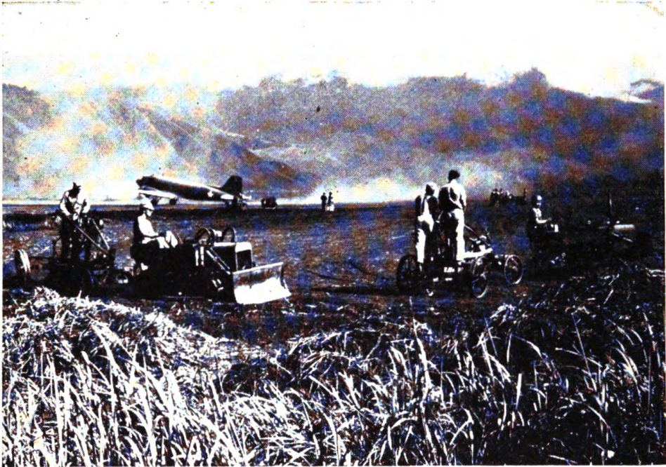
Figure 8. Grading an advanced landing field.
